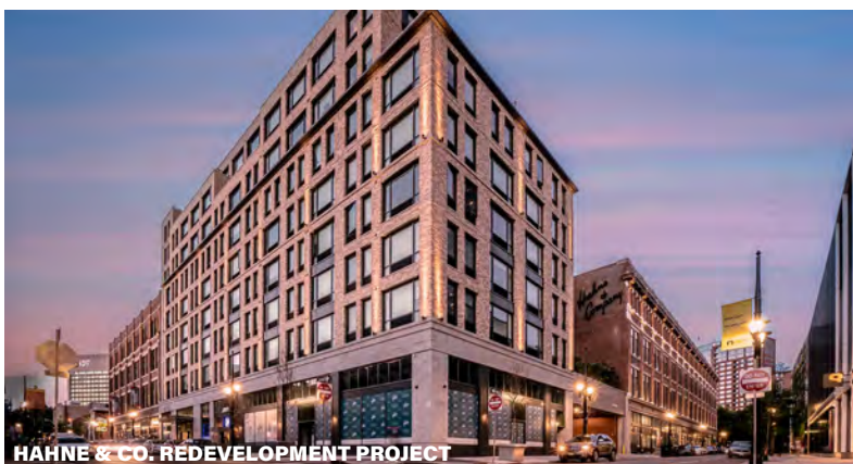
HAHNE & CO. REDEVELOPMENT PROJECT
